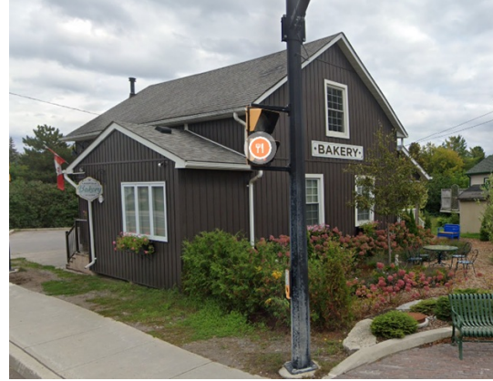
Photo of Lakefield Bakery (127 Queen Street, Lakefield) after exterior renovation work
