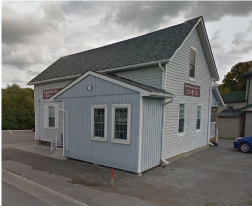
Photo of Lakefield Bakery (127 Queen Street, Lakefield) before exterior renovation work
