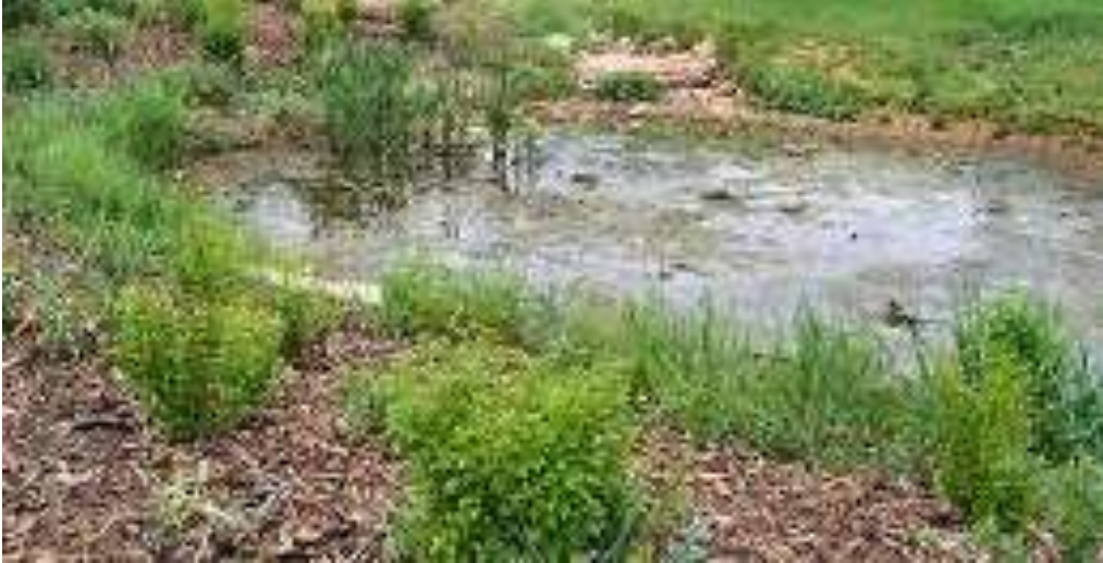
Typical subdivision stormwater pond
