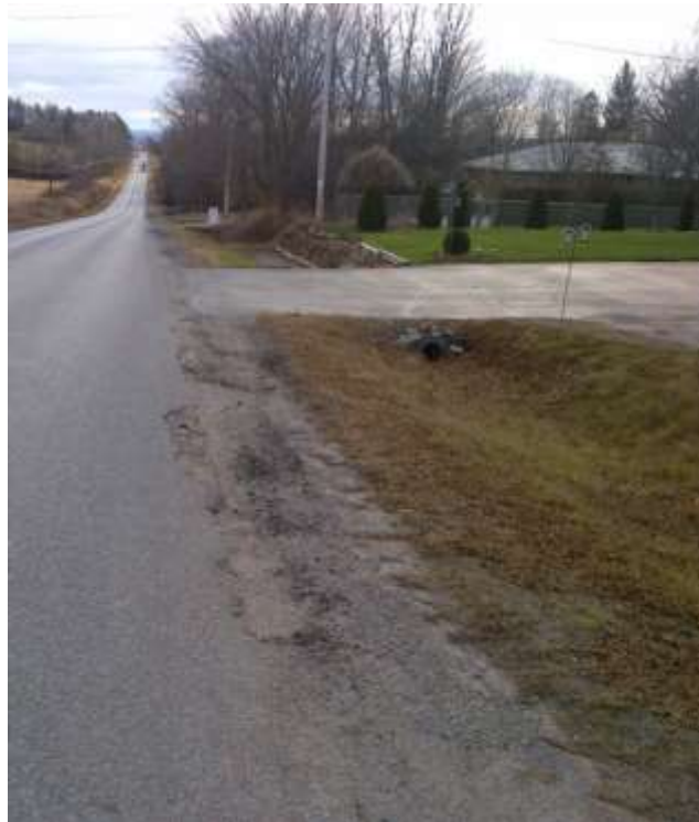
Rural road with open ditch drainage and tar & chip surface
