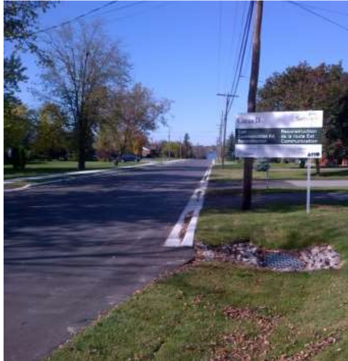
Urban road with curb & gutter, storm water and asphalt surface
