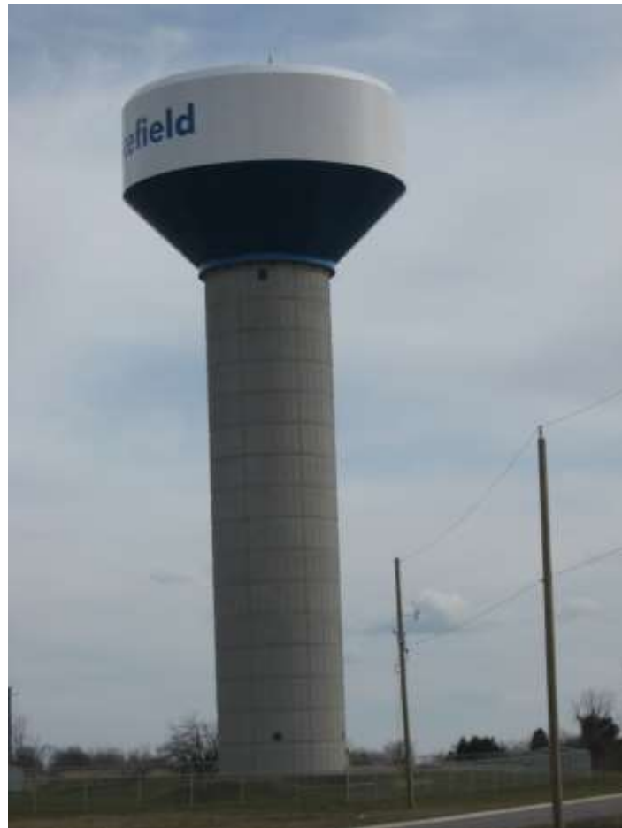
New water tower
