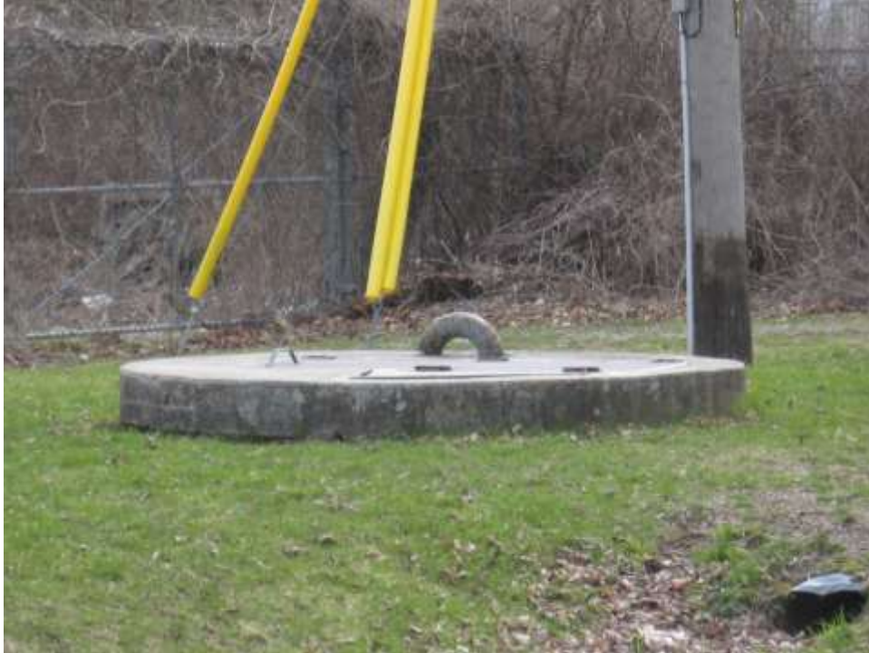
George Street Pumping Station Access
