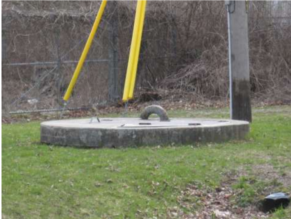
George Street Pumping Station Access
