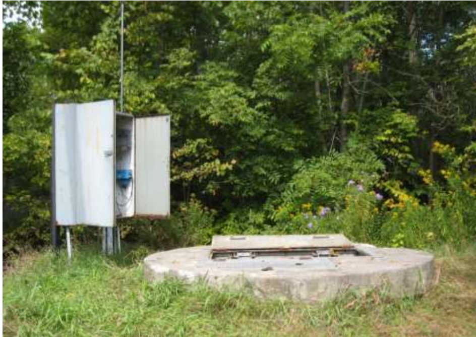
Lakefield College School Pumping Station Access
