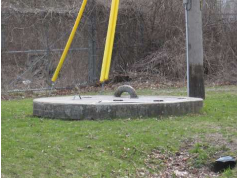
George Street Pumping Station Access
