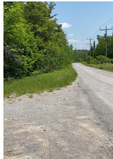
Photo 7: Looking east along Hillis Road from the site entrance (to the left in the photo); no roadside ditch was observed for Hillis Road.
