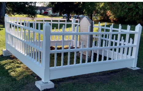
With Council approval, local craftsman Kent Wilson restored the historic Johnson Bickell Cemetery fence at Lakefield Road and the 6th Line, replicating 19th-century details using traditional joinery and locally sourced lumber.
