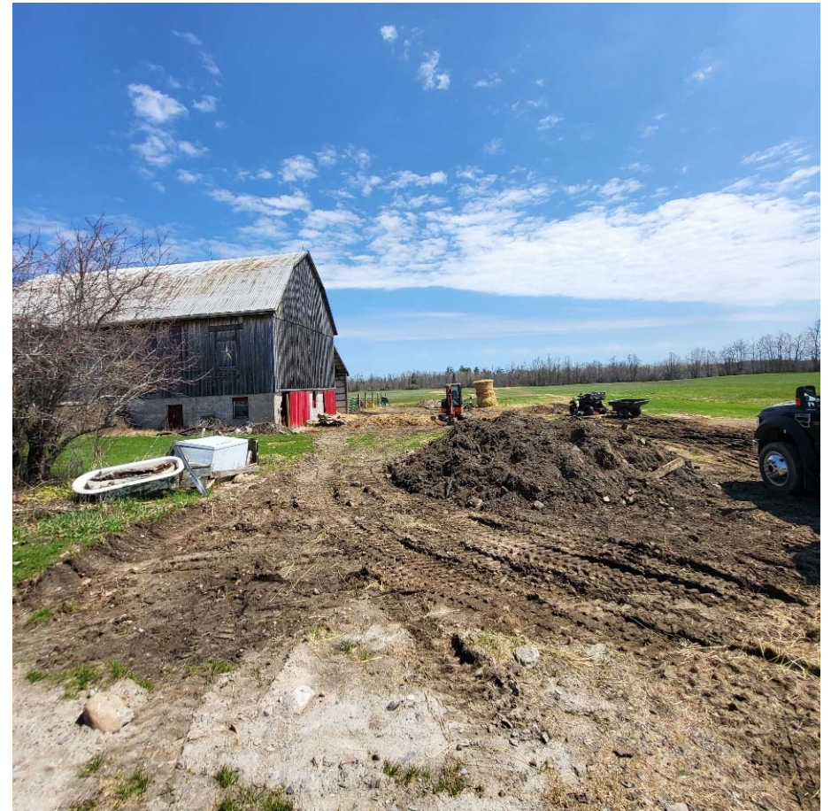
Existing barn – East view
