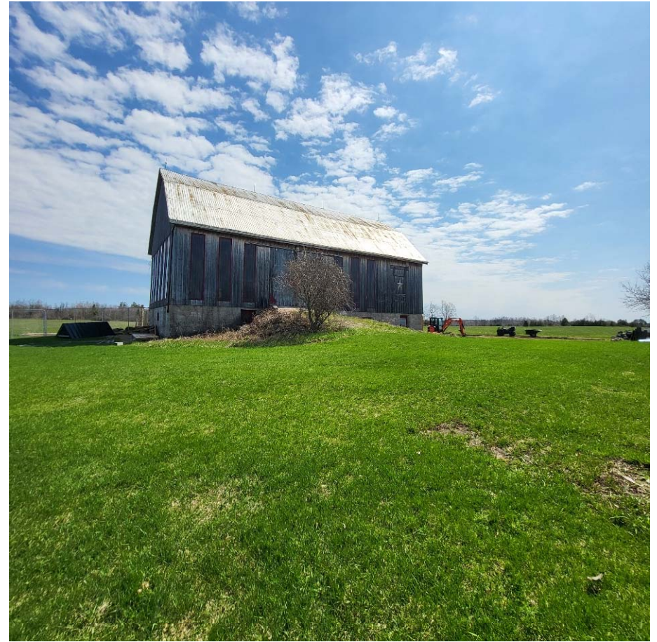
Existing barn – East view
