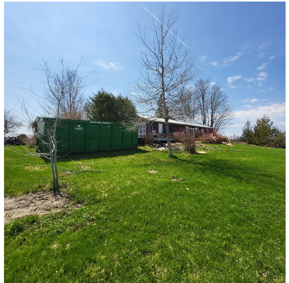
Existing dwelling – South-west view
