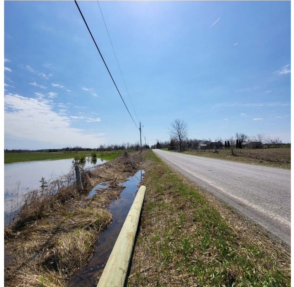
Northeys Road – South view
